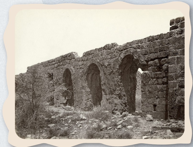
Photograph taken by Corporal Henry Philips R.E. in 1867 of an aqueduct bridge over the Wadi Nueima (PEF-P-827; Courtesy Palestine Exploration Fund)
